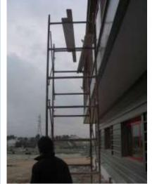
Maintenance personnel usually use substandard scaffolding especially when the works to be performed are short in duration or of "common nature".
