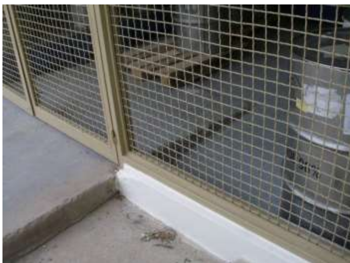
Secondary containment of the same area.
