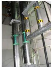
Well demarcated fluid-flow lines that facilitate identification as well as safe maintenance since it makes line-breaking easier and quicker to apply.
