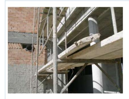
Scaffolding board used as a "supplement" to cover the working surface opening
